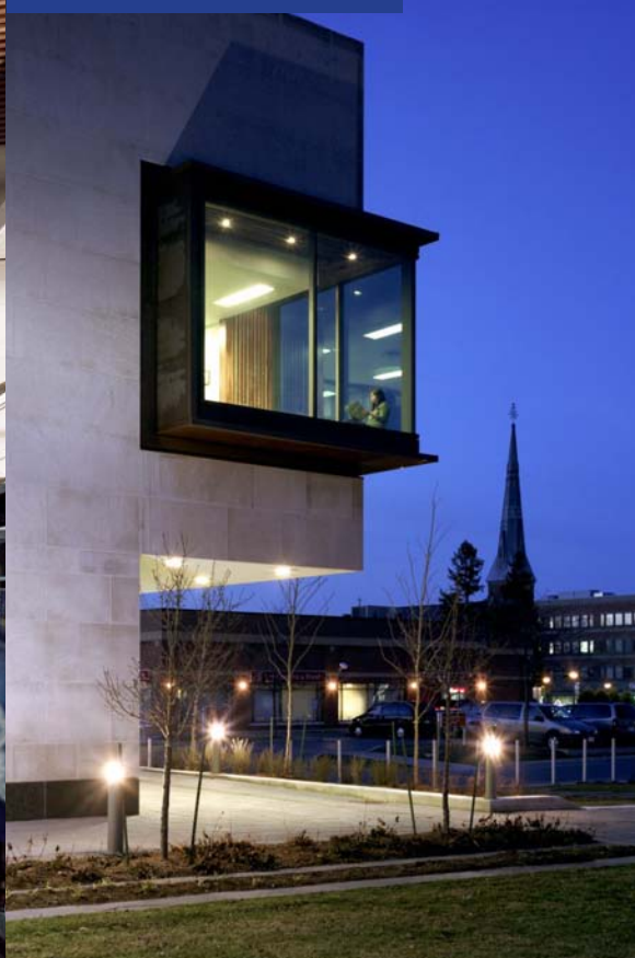
Whitby Public Library: Exterior Showing Adjacent Structures
