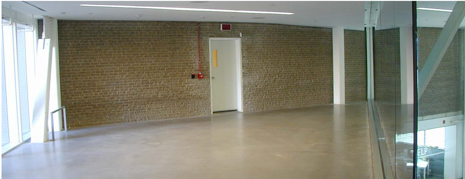
Areas that were slated for renovation on the 3 rd floor of the Library Building
