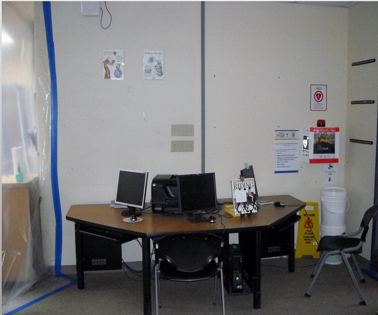
Computers station before/during remediation.
