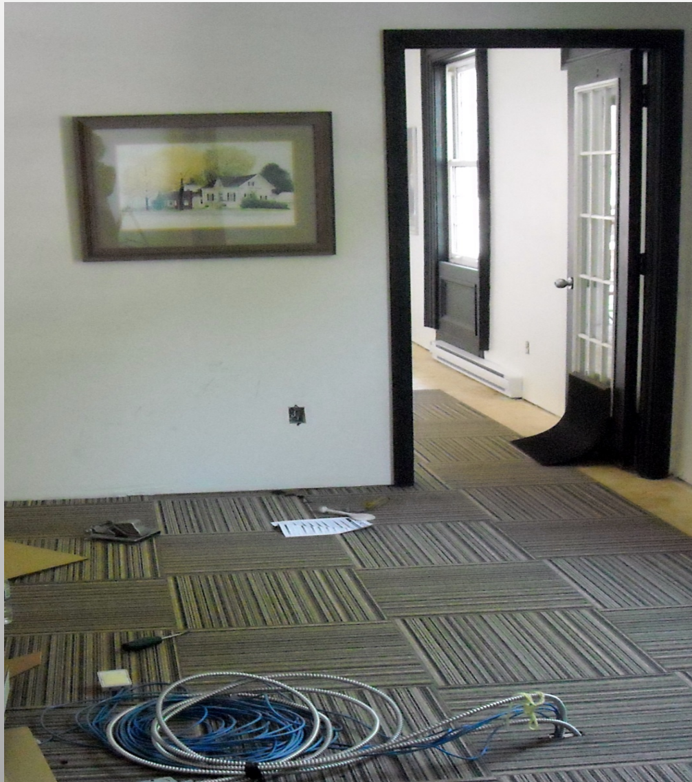
Carpet was finally installed in the backroom.
