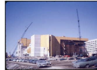
Scott Library - showing yellow insulation cladding under precast Source: https://digital.library.yorku.ca/yul-1121744/new-object
